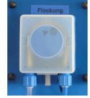
Figure 13, Flocculant dosing pump
